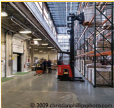
The Yawkey Distribution Center, a 117,000 square foot building for the Greater Boston Food Bank's food distribution programs.
